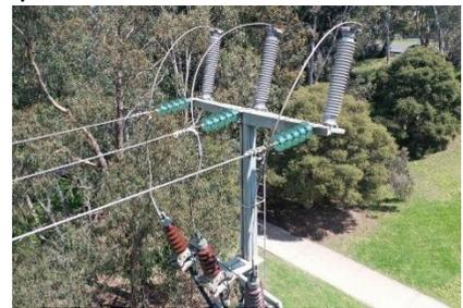
The poles under assessment provide critical oil filled cable Underground to Overhead (UGOH) connections for parts of Geelong and Melbourne so their detailed assessment, and the timing of the project to align with seasonal demand was critical.
